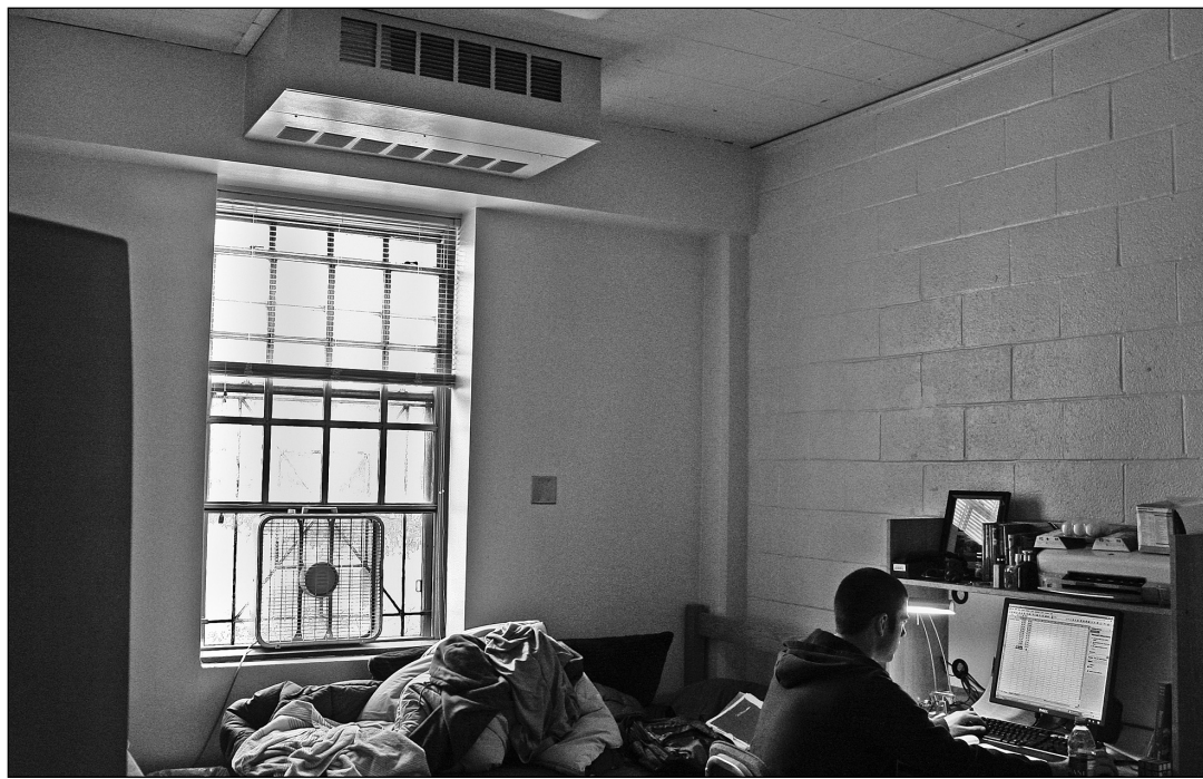
Two prototype dorm rooms have air conditioning units mounted on the ceiling and special insulation on one of the walls.
